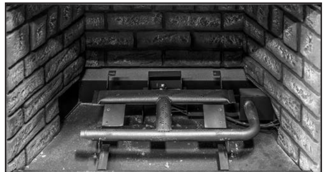
Figure 38: Remove the 6 screws highlighted in figure 37 using a Torx T-20 screwdriver and remove the air deflector
