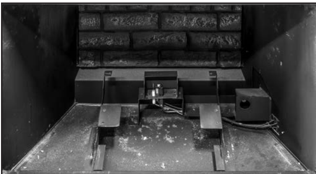
Figure 39: Lift the burner off the mounts and pull it out of the inlet box. The unscrew the panel brackets (T20's) from each side of the baffle to remove the left and right side liners.
